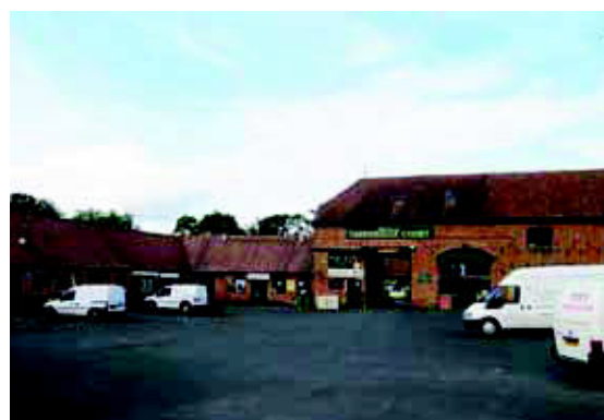
Tardebigge Court, Hewell Lane
