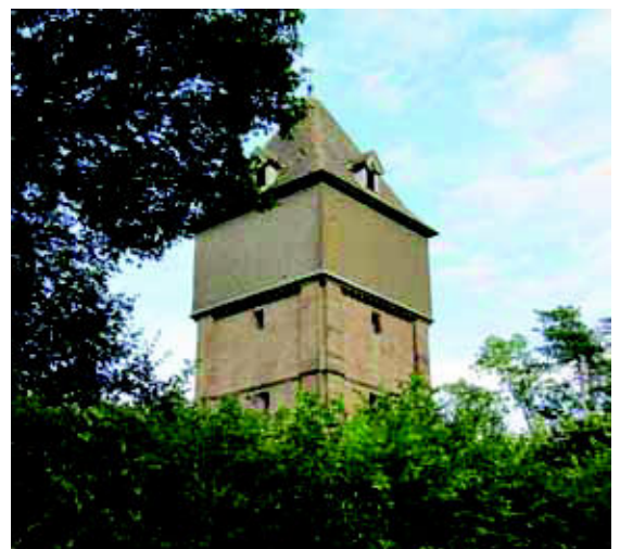
View of water tower from Hewell Lane
