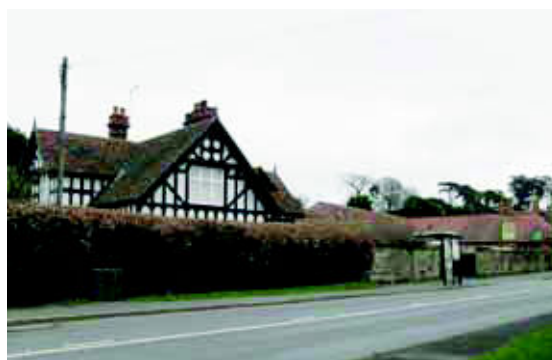
Dairy Cottage and Tardebigge Court
