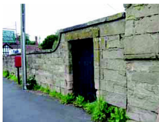
Wall to Tardebigge Court
