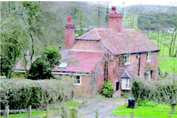
Old Papermill Cottage, off Hewell Lane
