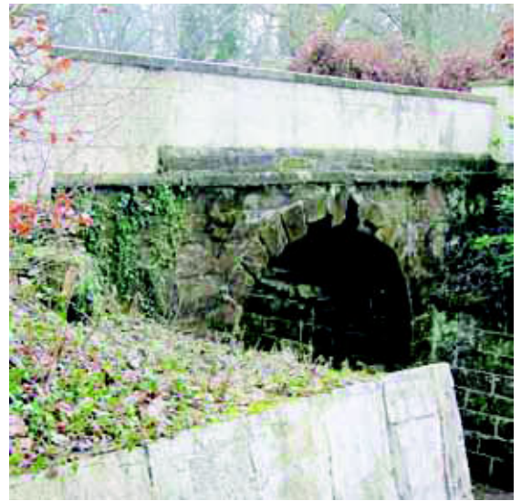
Sandstone bridge, Hewell Park
